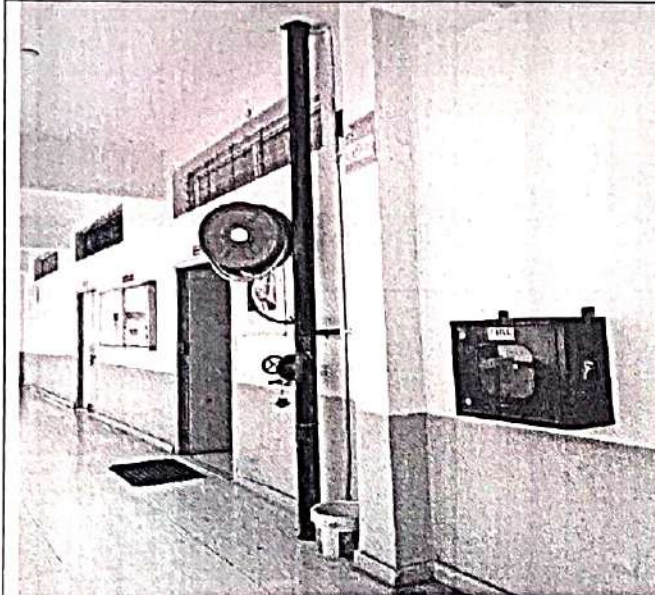
Fire safety Measure
